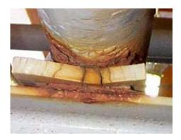
Figure 2.3. Crevice corrosion between pipe bottom and pipe support [6].
